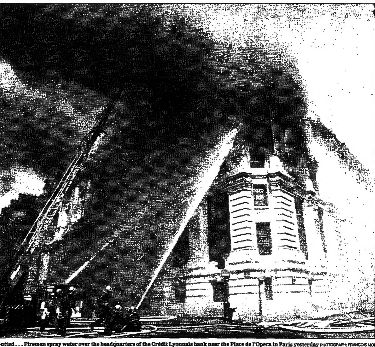
Gutted... Firemen spray water over the headquarters of the Crédit Lyonnais bank near the Place de l'Opera in Paris yesterday. PHOTOGRAPH: FRANCIS MOR...
